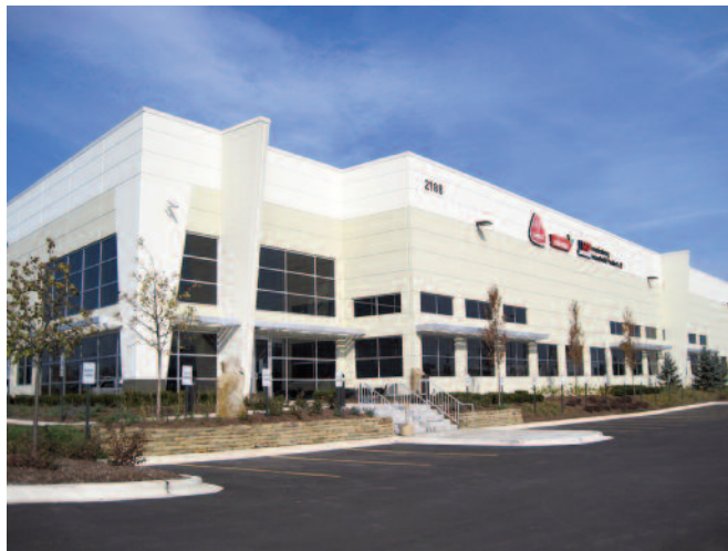
FHP North America Headquarters
