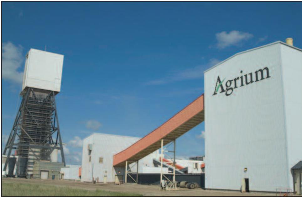
Agrium's potash production facility in Vanscoy, Saskatchewan
